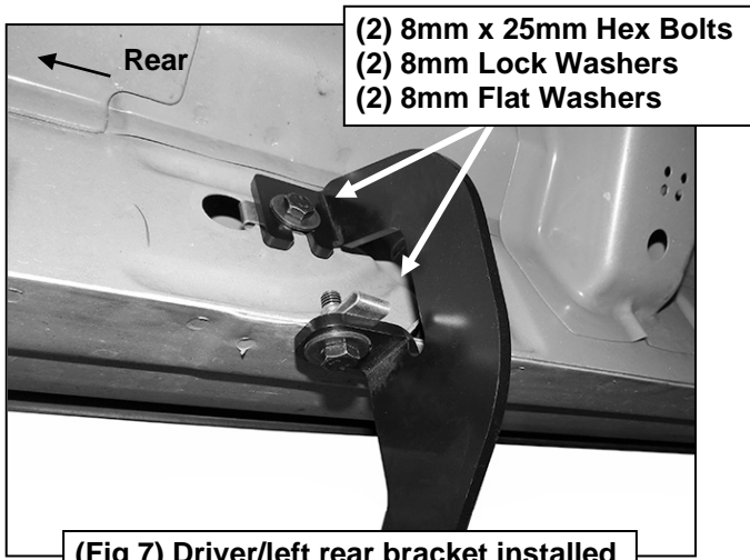
(Fig 7) Driver/left rear bracket installed
