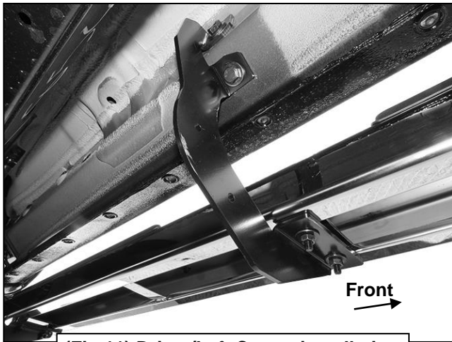
(Fig 11) Driver/Left Center installation
