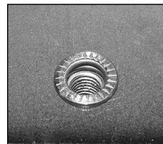
(Fig 6) Example of fully installed 6mm Insert
