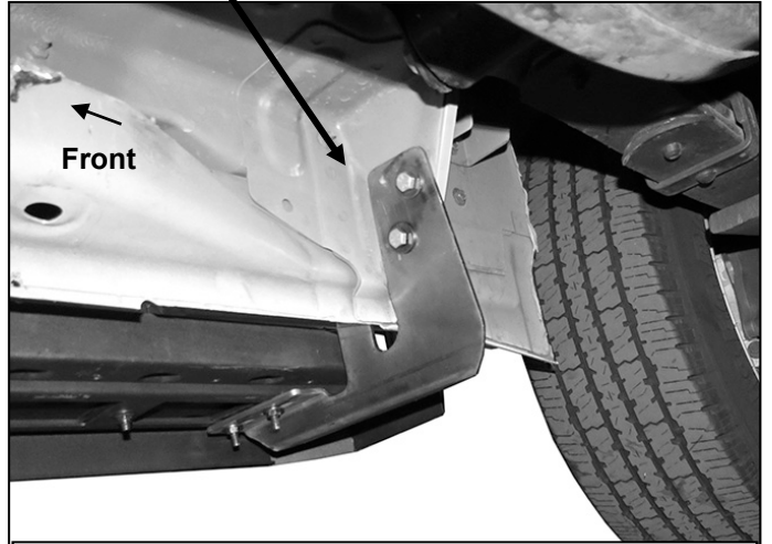
(Fig 20) Passenger/right rear complete installation
