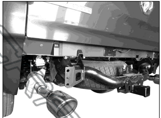
(Fig 4) Factory bumper assembly removed
